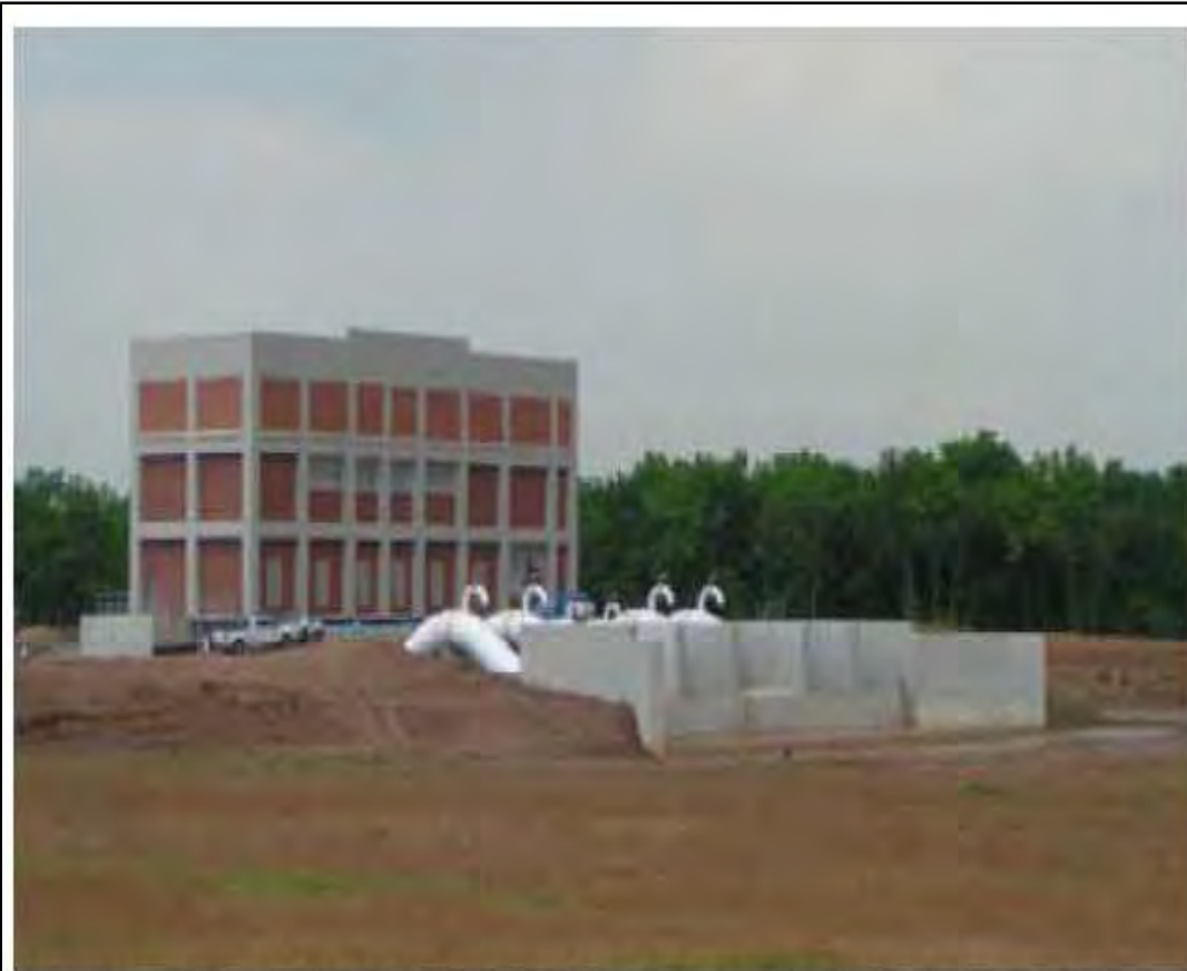
Construction of Pump Station No. 1 (Front/outlet side view)
